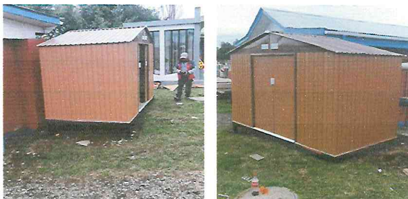
BODEGA CEMENTERIO MUNICIPAL TEODORO SCHMIDT
